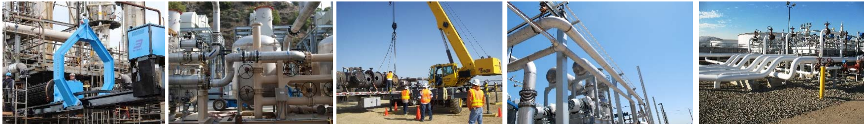
Mechanical maintenance services, primarily piping, electrical & instrumentation maintenance, engineering, small capital construction and turnaround support services
