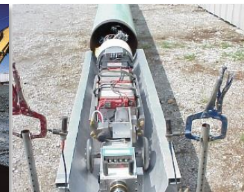
Robotic Interior Weld Coating
